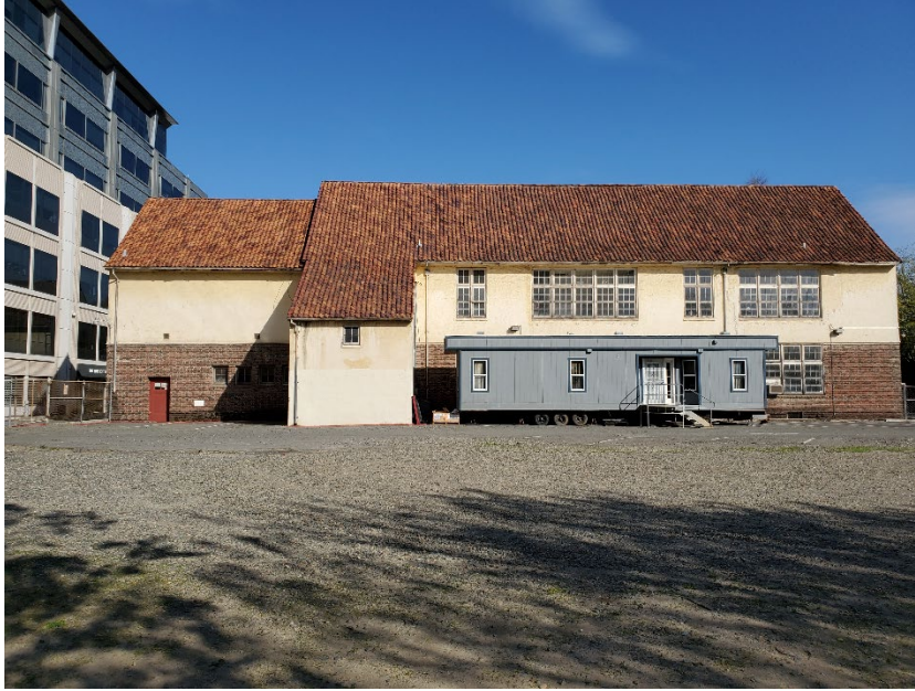
Photo 21 Northwest façade, camera facing southeast
